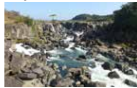
① Sogi Waterfall Diversion Channel
